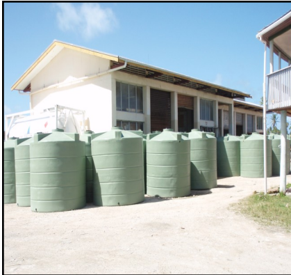
Rota Water Tanks
