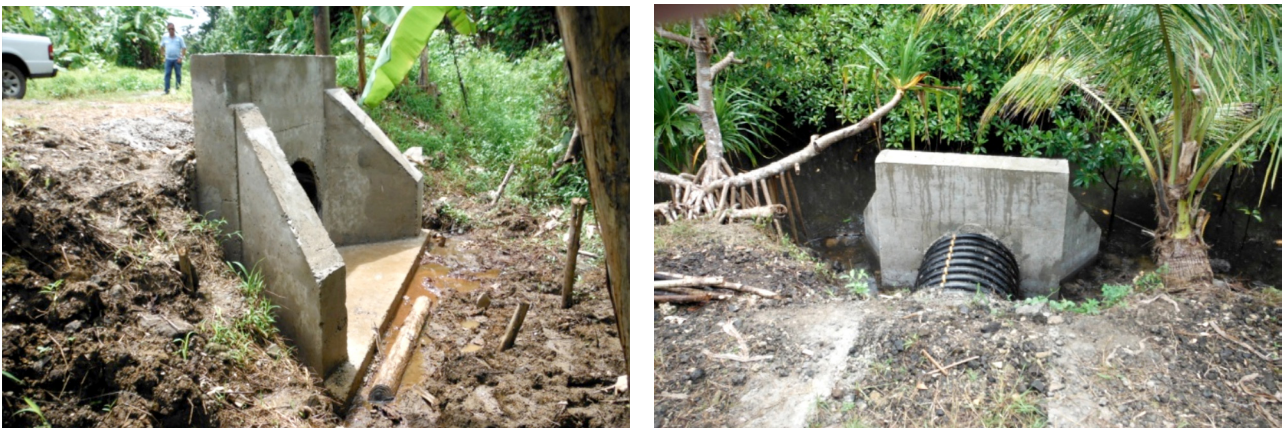
Figure 4. New culverts installed by the project.
