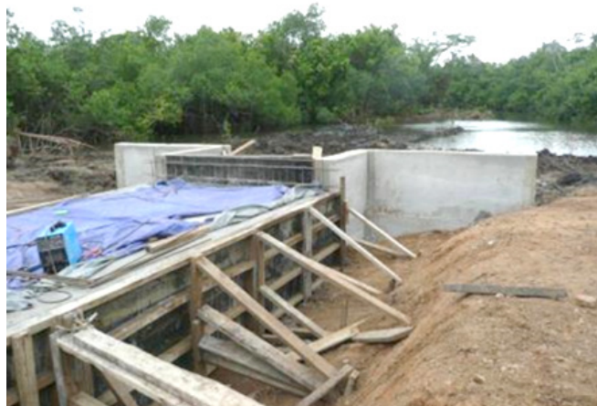
Figure 7. Installing the tide gate at Waikete.
