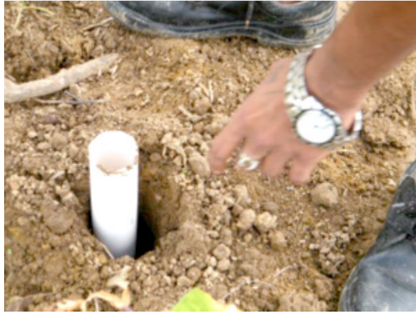
Figure 5. Installation of piezometers for measurement of water table.
