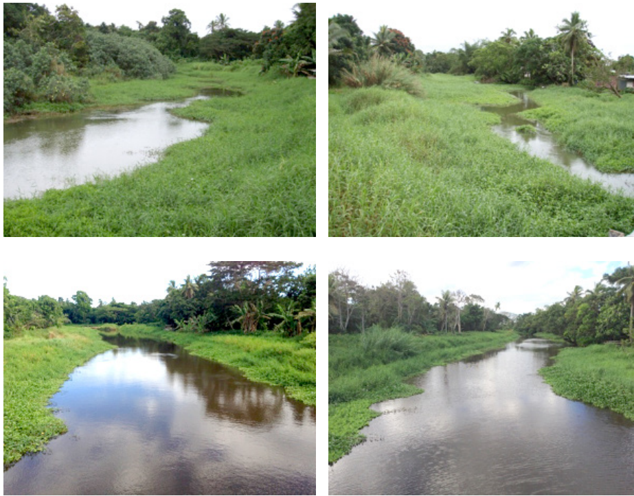
Figure 6. Qaraniki Creek at Vunivaivai bridge before (top) and after dredging (bottom). The images on the left hand side are looking downstream (east) from the bridge, and on the right upstream (west).
