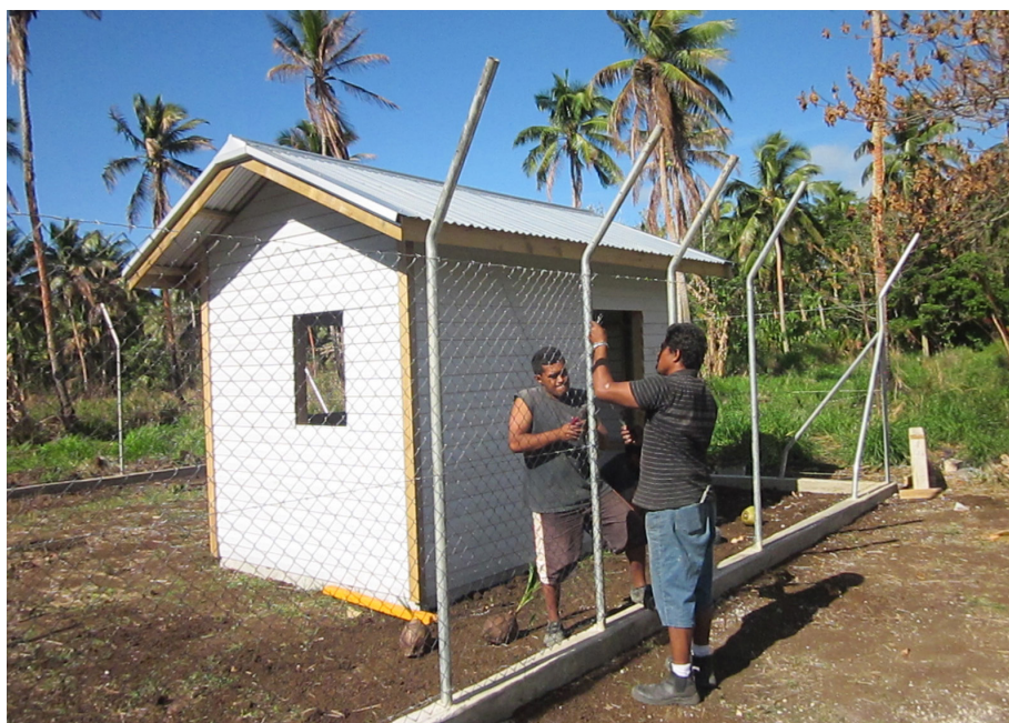
Figure 5. Securing one of the new pump houses.
