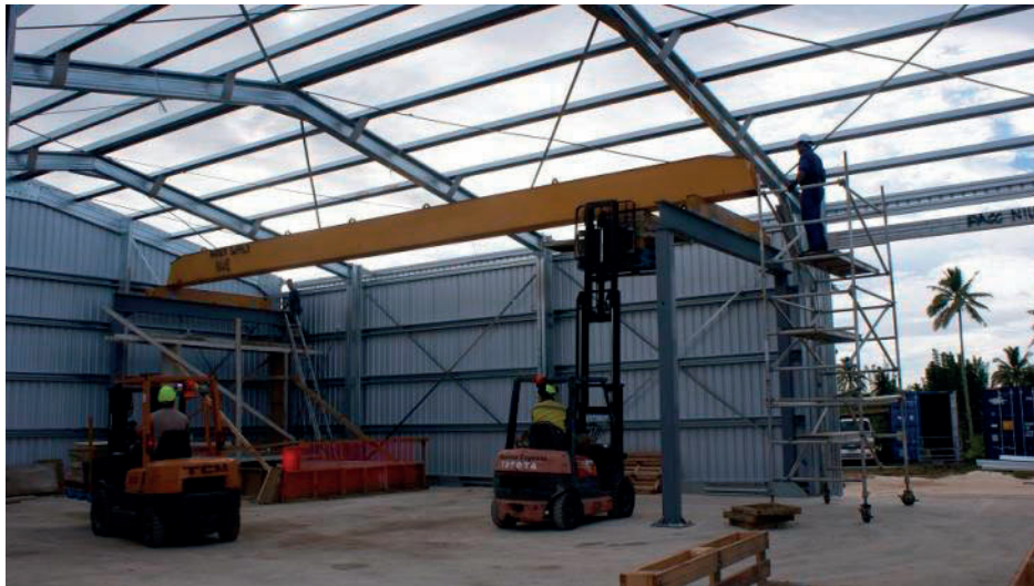
Figure 14. Building the shed. (Photo: Niue PACC Project.)
