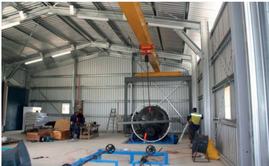
Figure 15. Installing the moulding equipment. (Photo: Niue PACC Project.)
