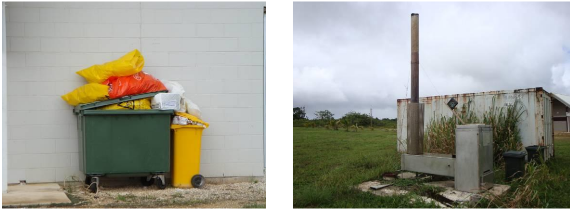
Picture 4: Medical waste storage and incineration at Niue Fooo Hospital
