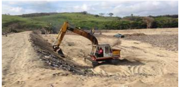
Improvement of Disposal site, Sigatoka Town
