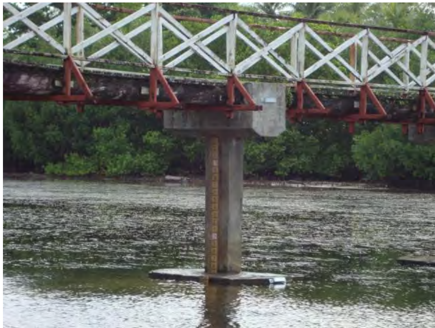
Figure 2-11: Walung Bridge reference staff gauge, and mounting brackets for PVC pipe and housing.
