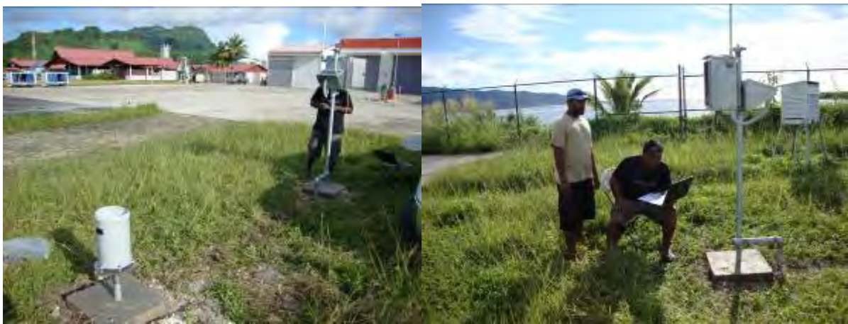
Figure 2-1: Installed rainfall and solar radiation station at Okat airport.
