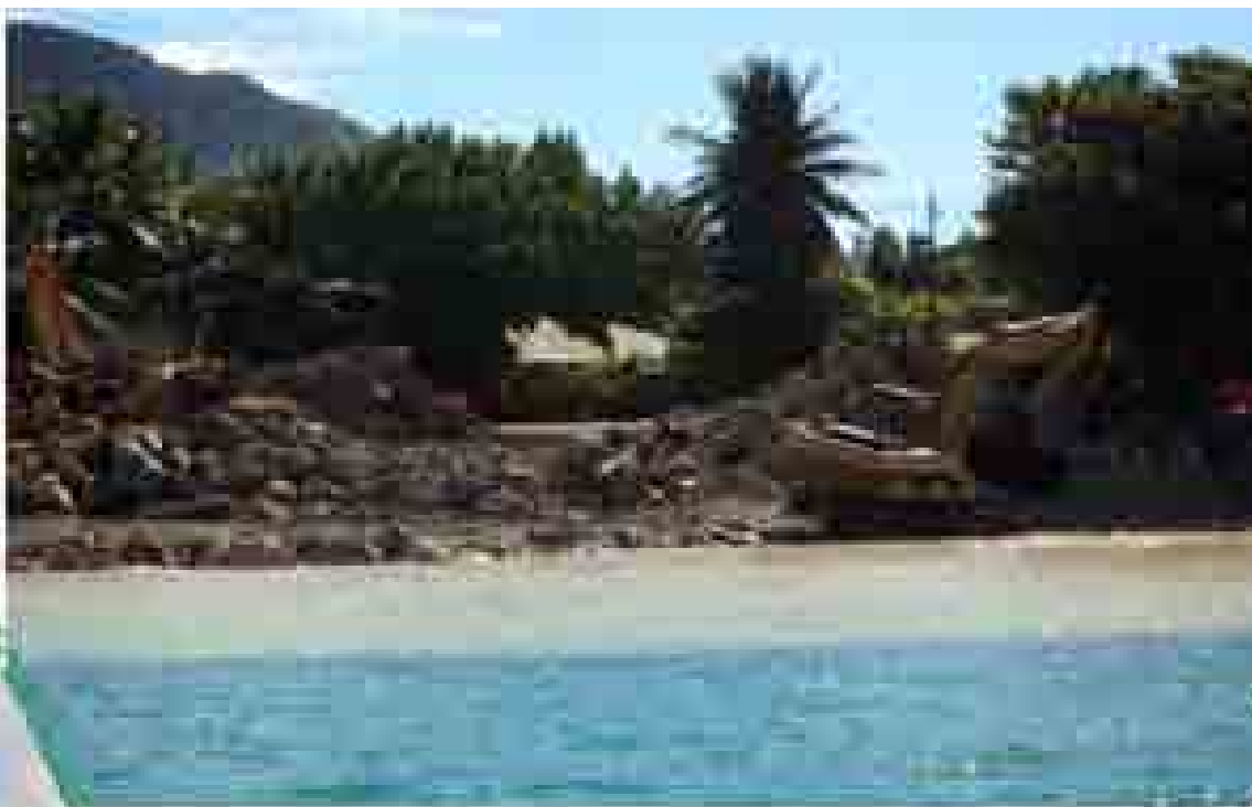
Harbour Construction, Avatiu, Rarotonga
