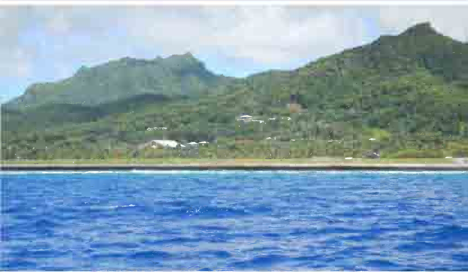
Seawall, Nikao, Rarotonga
