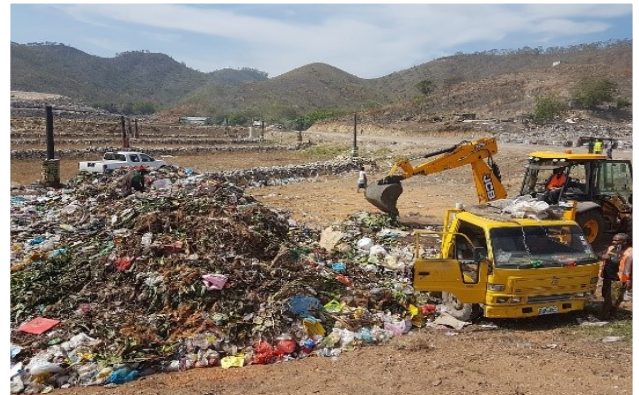
First landfill operation at Cell 1
