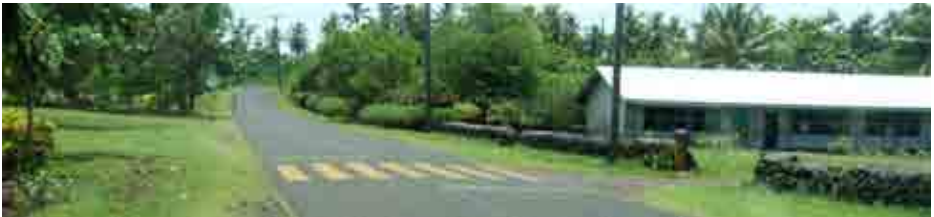
Main road crossing near school
