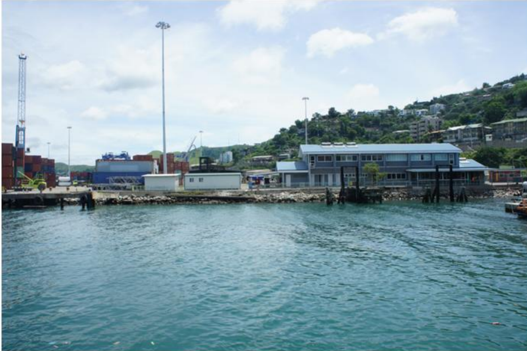
Figure 4: Eastern view of Laurabada Wharf, Container Terminal, PoM
