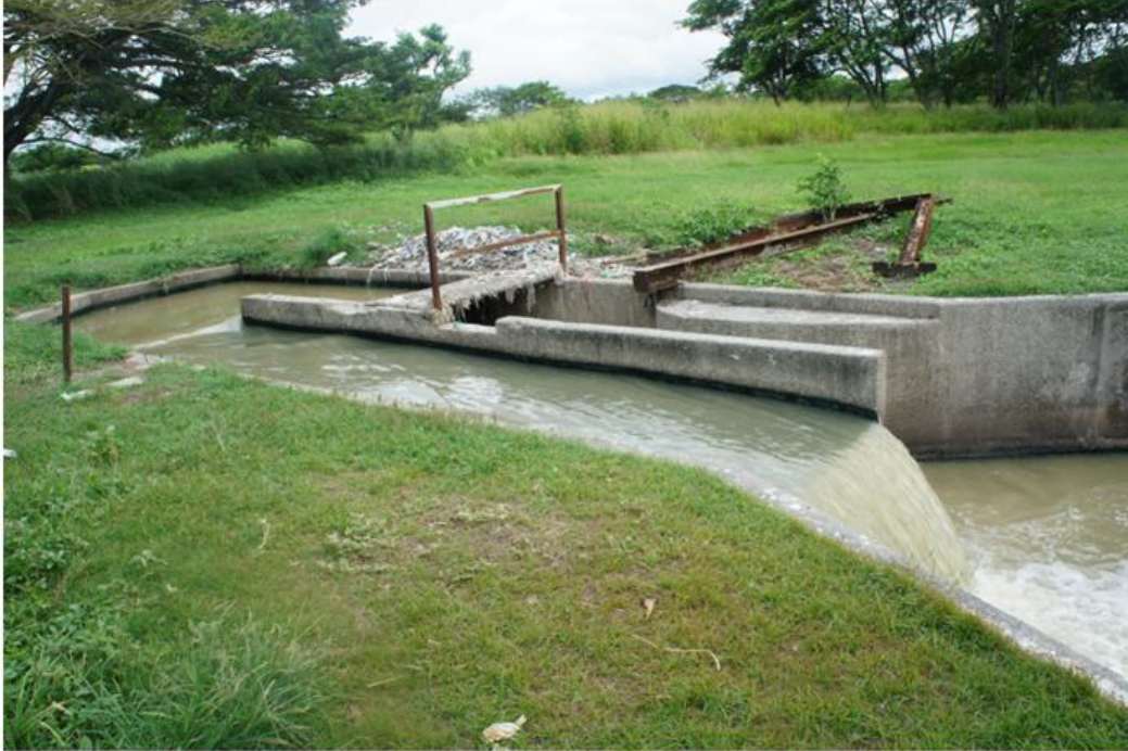
Figure 7: SW view of Port Moresby City's sewage settlement pond's inlet
