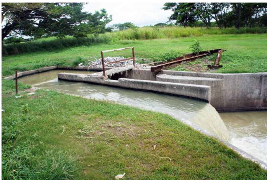
Figure 8: SW view of Port Moresby City's sewage settlement pond's inlet
