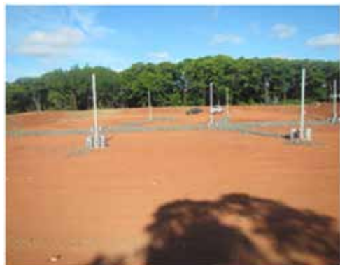
Rehabilitated Cells with Installed Gas Ventilation and Leachate Facilities
