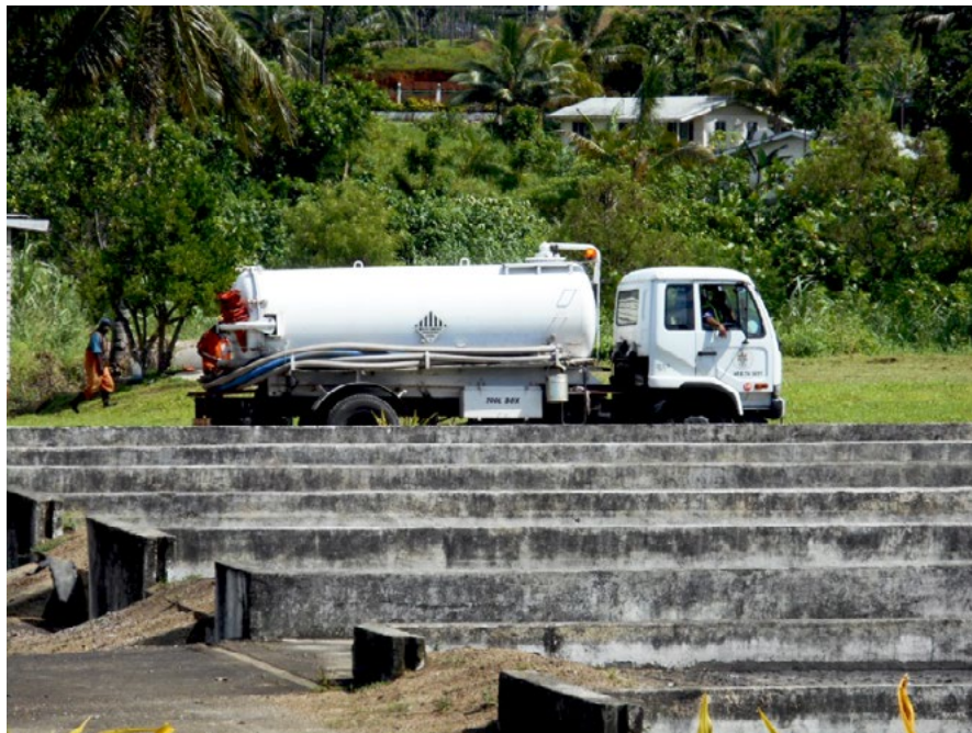
Tanker truck discharging at WAF wastewater treatment plant
