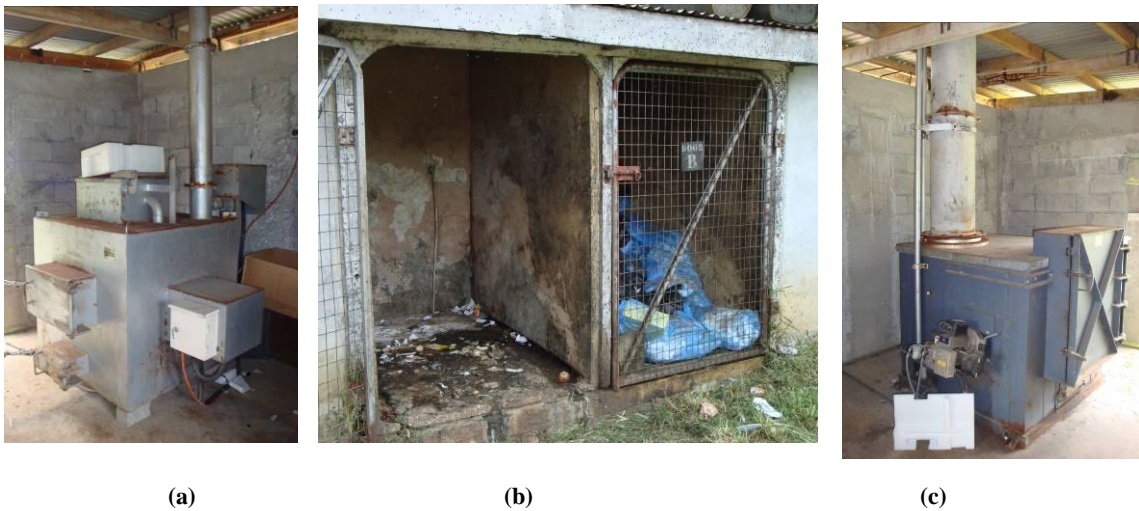
Figure 2: (a), (b) Incinerators located at the Port Vila Central Hospital; (c) medical waste storage area
