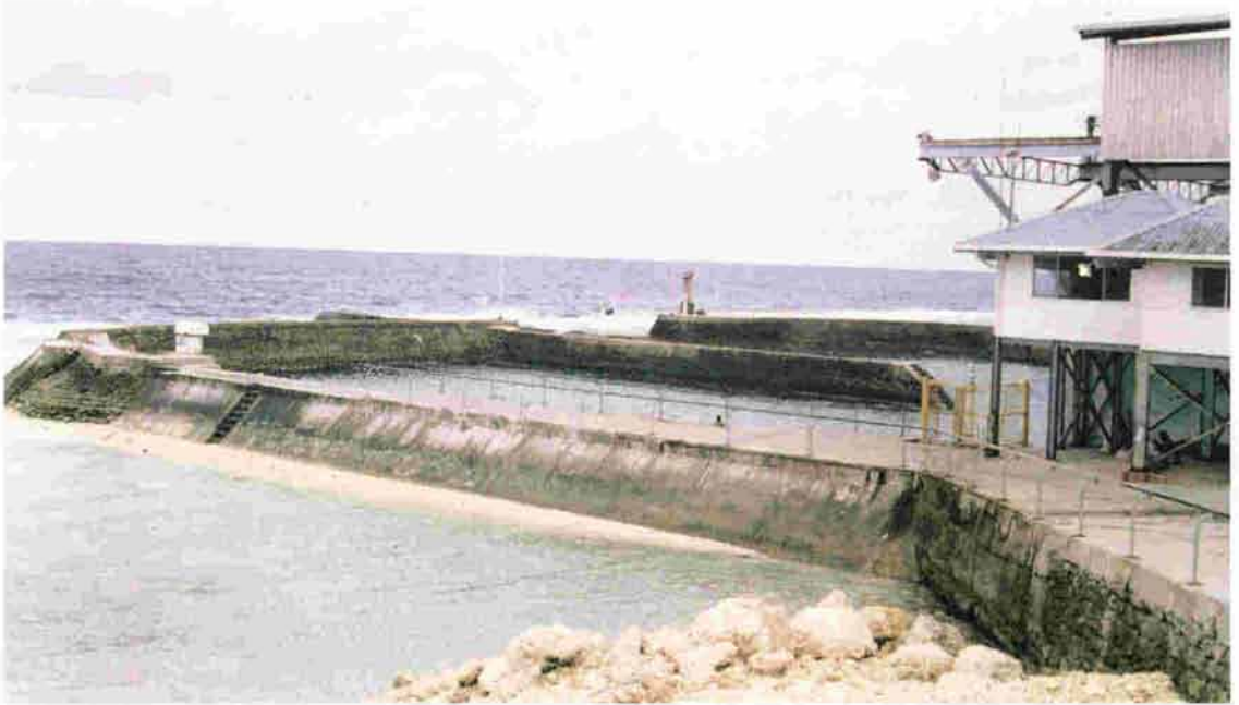
Nauru's harbour sea wall protects SPREP's tide gauge, set in front of the harbour buildings. An earlier NOAA gauge rests on the outer sea wall.
