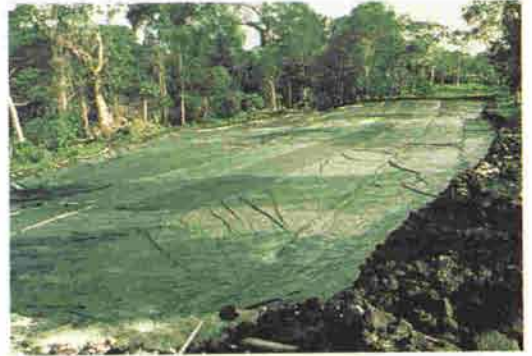
Environmental Impact Assessments for development projects such as roads should be carried out as part of project planning – not after the fact!
