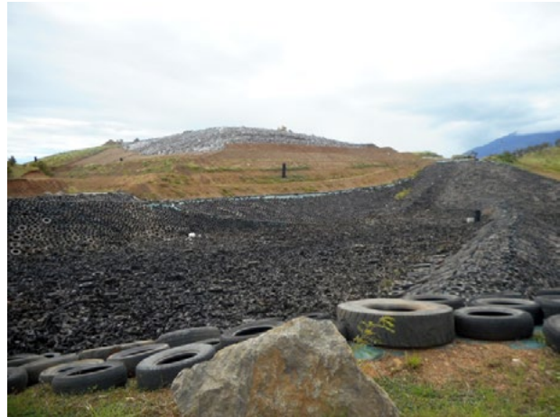
Figure 6b: CSP landfill – new area with recycled tyres as drainage
