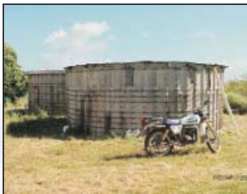
Water Tanks in Aitutaki.
