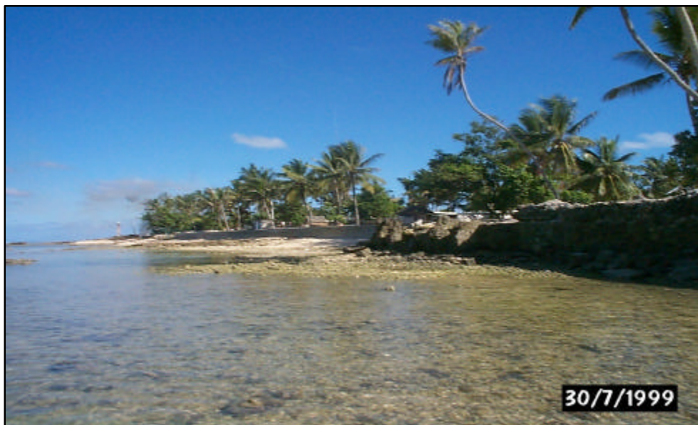
Figure 5.2. Seawall construction in Tarawa, Kiribati.
