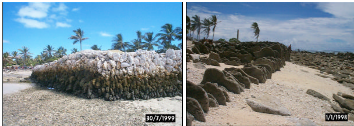
Figure 5.9. Interlocking coral rubble seawalls along the coast in Tarawa, Kiribati.
