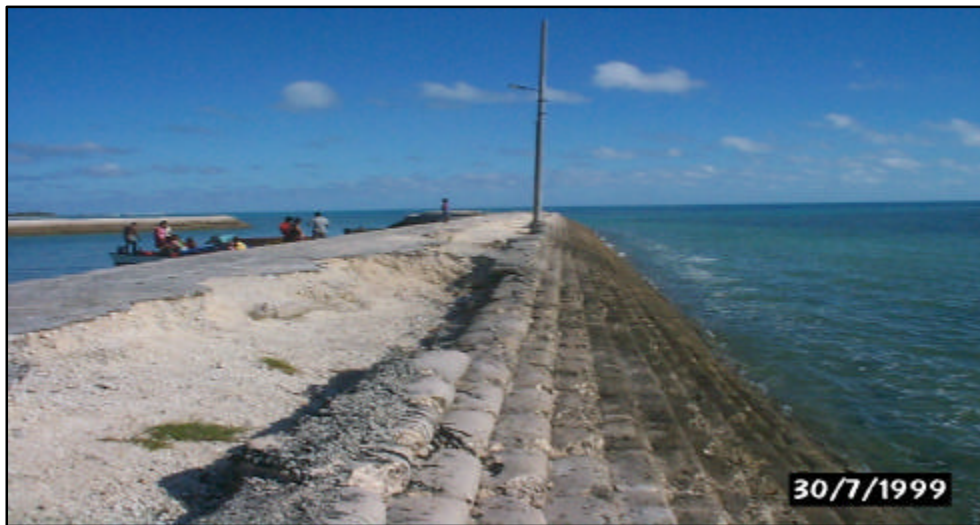
Figure 5.1. Breakwater construction in Bairiki, Kiribati.
