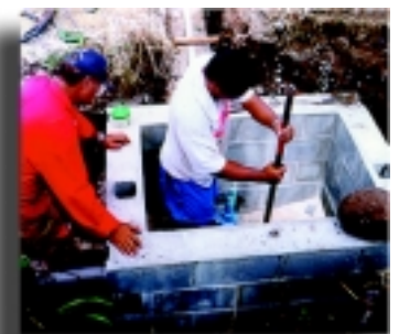
Rarotonga water supply system...man at work.
