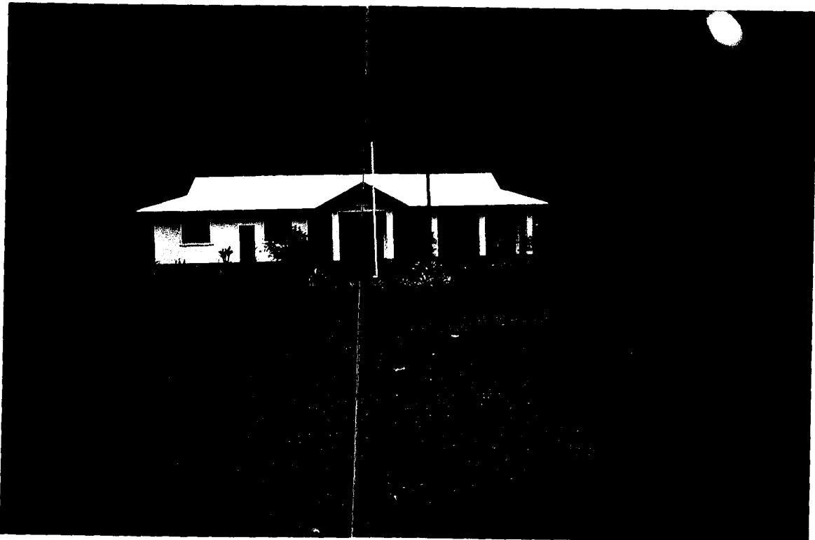
Photo 12 Courthouse at Sola on the island of Vanua Lava where the Torba Province is administered.
