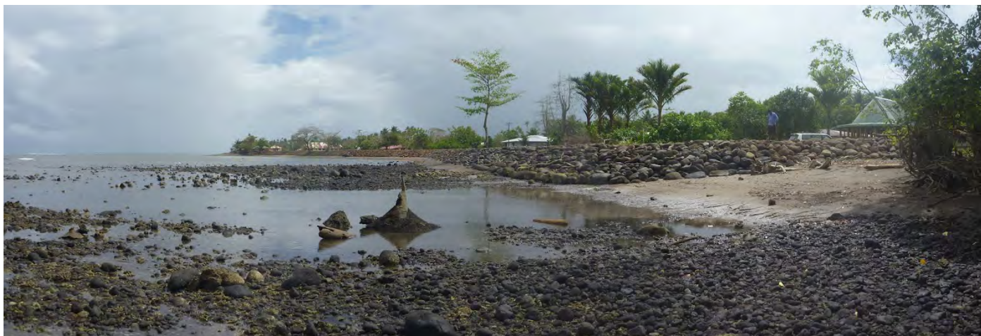
The construction of a seawall in Tafitoala is an example of coastal protection. Photo: Gabor Vereczi
