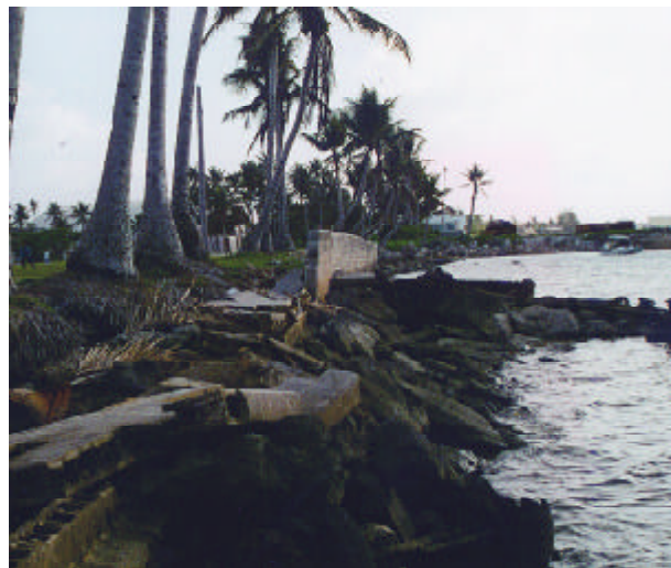
Rising sea level in Majuro, Marshall Islands is damaging the sea walls erected to protect the islanders
