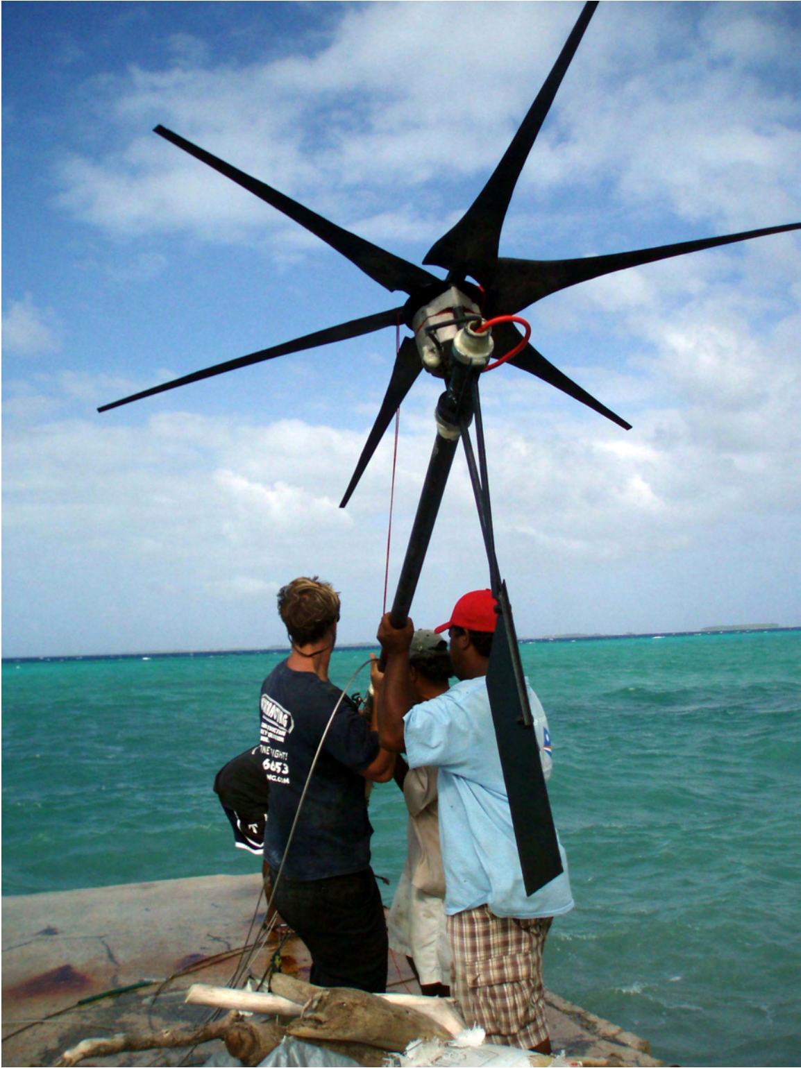
Figure 4. Installing the replacement windmill.
