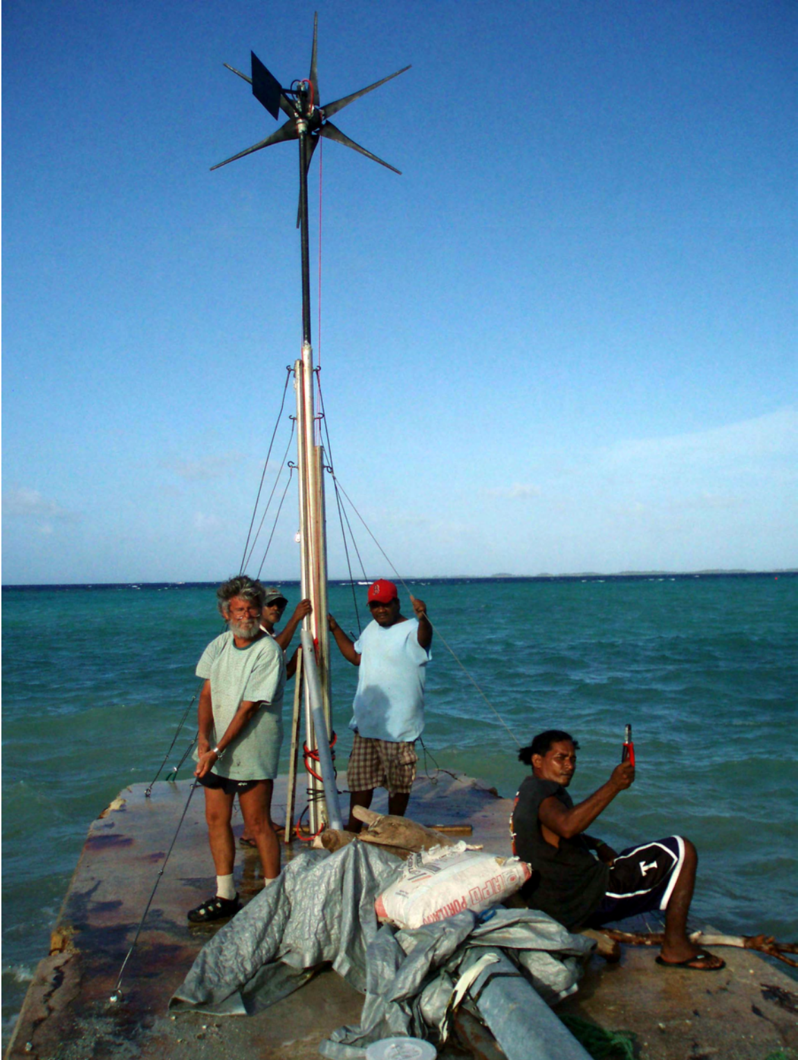
Figure 5. The windmill in place with guy wires attached.
