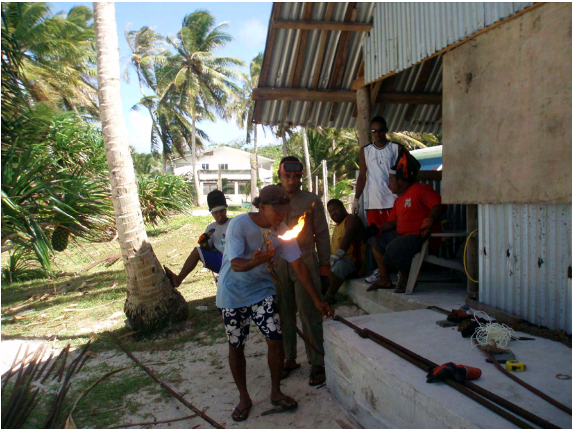
Figure 2. Workshop facility constructed at Jabo Village, Arno. Katwel Jormelu is shown training the local team in use of a gas torch to bend steel bars to make Biorock shore protection modules.
