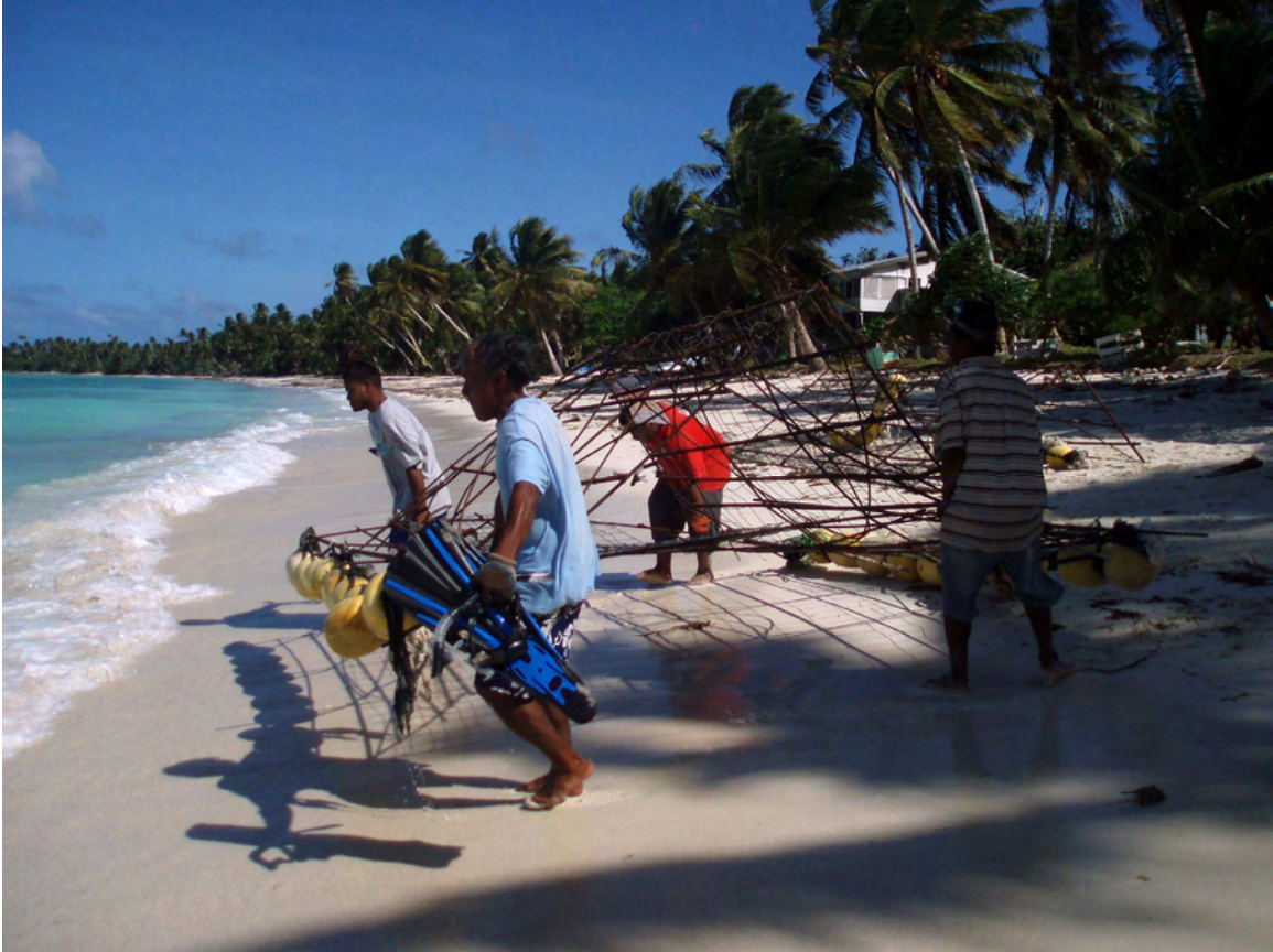
Figure 12. Transporting a shore protection module from Jabo Beach.
