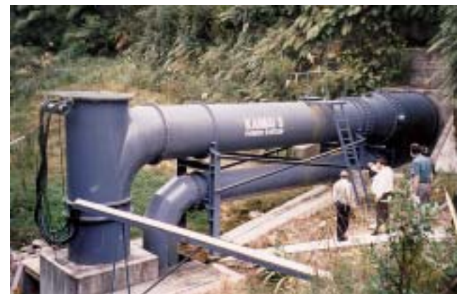
A diverted stream powers a turbine to generate electricity
