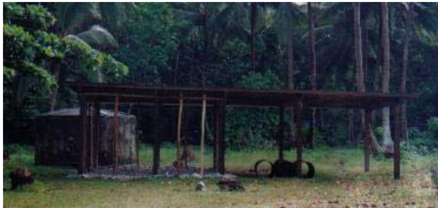
Fig: 7. One of three rainwater catchment and storage facilities
