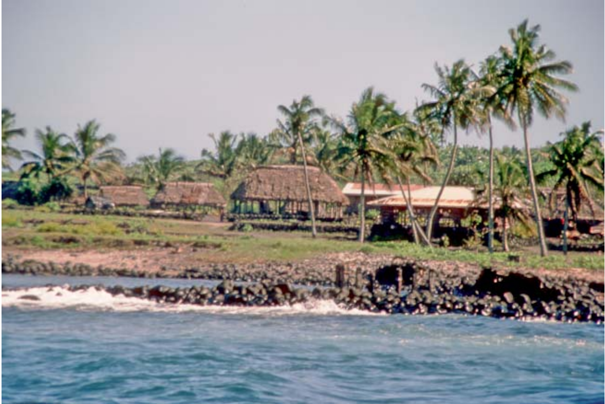
Figure 9 Samoan fale on the island of Savai'i. Note that these buildings have hipped roofs and are placed on significant mounds.
