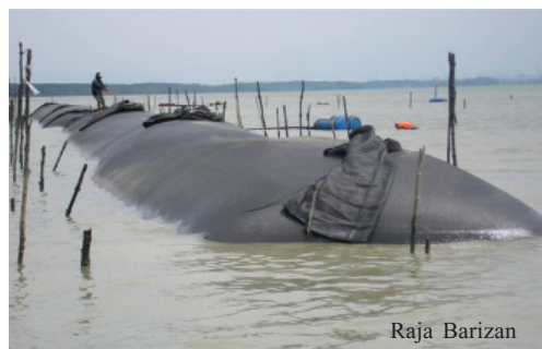
Fig. 13. Rock revetments constructed to safeguard against coastal erosion (L) Fig. 14. Sand-filled geotubes constructed to protect eroding shores (R)
