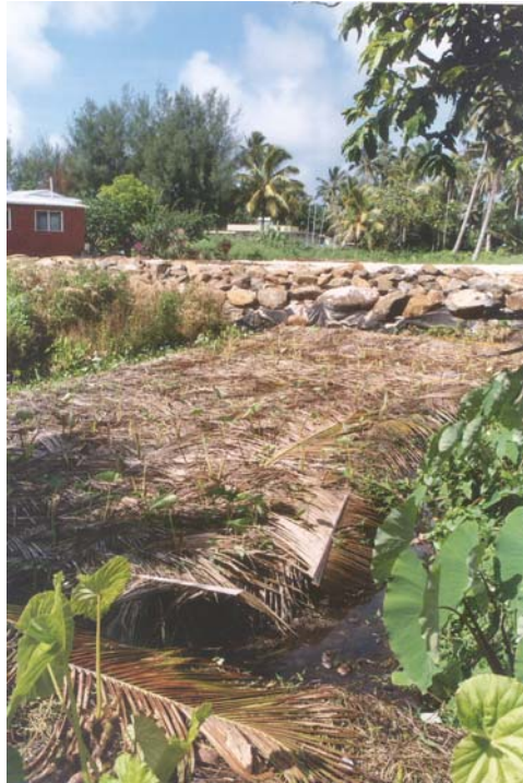
Plate IX: Example of a wetland area that has been partially reclaimed using boulders and sand (see rear of photo). This area has been reclaimed for the construction of tourist accommodation. The area in the foreground is some of the remaining taro swamp
