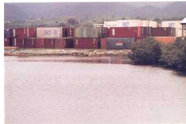
Plate 35. A seawall built to protect this reclamation close to the Port of Suva, Fiji, has failed after a short time. The mangroves that were cleared from the site would have provided better protection.
