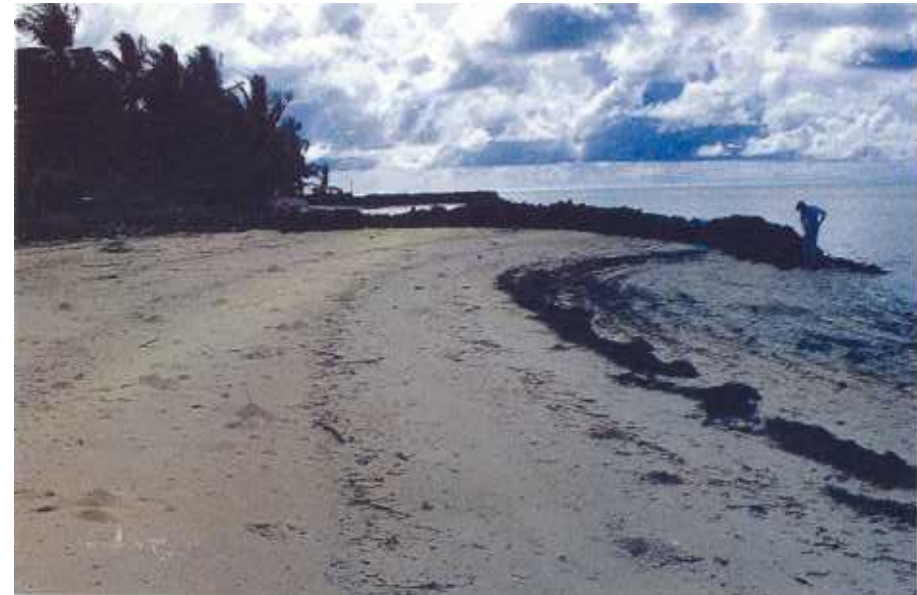
Plate 41. The groyne has been built out across the beach to trap sand prior to making a reclamation. Sand will be lost to the beach on the other side of the groyne, and beach erosion will take place.
