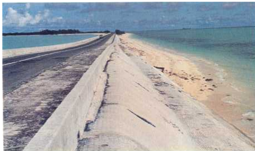
Plate 42. Concrete-filled mattress protection for the Nippon causeway in Tarawa, Kiribati, is designed to flex so that it will not fail as settlement takes place, but it is not suitable for exposed conditions.
