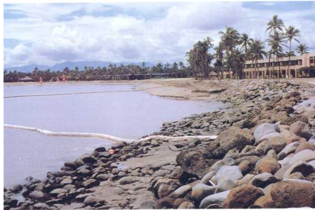
Plate 34. Artificial replenishment of beach in front of the Regent of Fiji is being carried out by trucking sand to replace that lost by erosion. The erosion problem was caused by a groyne which blocked off the natural supply of sand to the beach.
