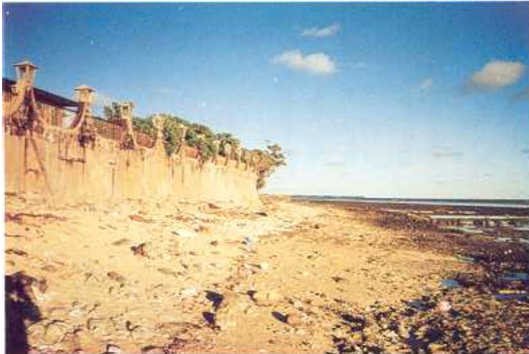
Plate 1. A rather elaborate vertical concrete block seawall protecting property on the ocean side of Majuro Atoll, Marshall Islands. Note the narrow reef flat, lack of sandy beach and the foundations of the seawall.
