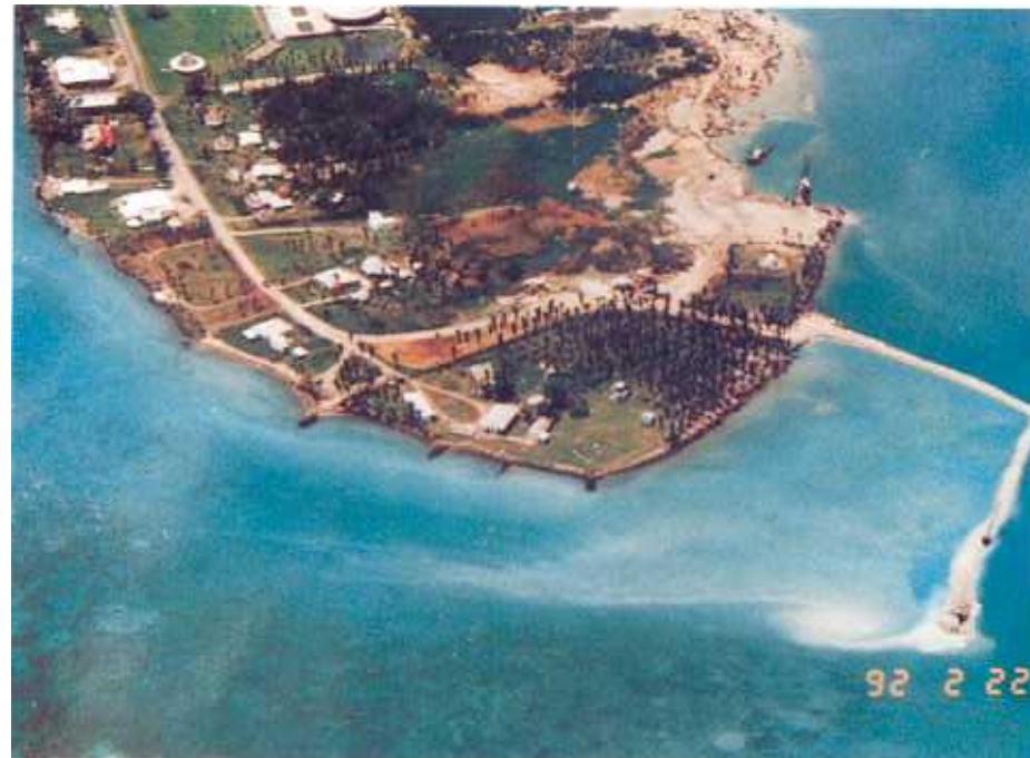
Plate 9. Foreshore development, groynes and dredging operations at Mulinu'u Point, Western Samoa, are affecting the natural movement of sand around the point. Note the small spit forming around the end of the dredging causeway, bottom right corner of photo.
