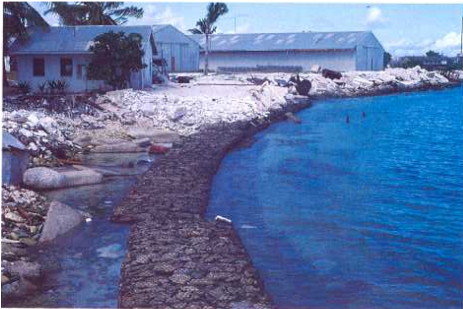
Plate 31. Erosion threatening government buildings on the ocean side of London, on Kiritimati (Christmas Island), Kiribati. Attempts to protect the buildings include dumping of large concrete slabs, junk vehicle parts and reno mattresses (a flat version of gabion baskets).
