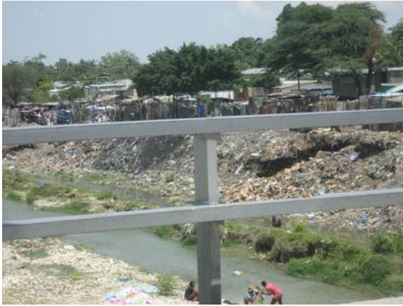
Poor, unregulated settlements on the river's edge in Haiti are highly prone to flooding. (Photo by Vincent Sweeney)
