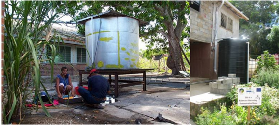
Rainwater harvesting such as on Banaba, Kiribati (l) and Mabouya Valley, Saint Lucia (r) has been under utilised in many small island countries. (Photos by Marc Overmars and Donna Spencer)
