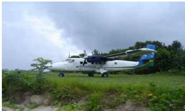
Picture 4: Coastal Erosion impacting on infrastructure - Fera airport, Isabel Province
