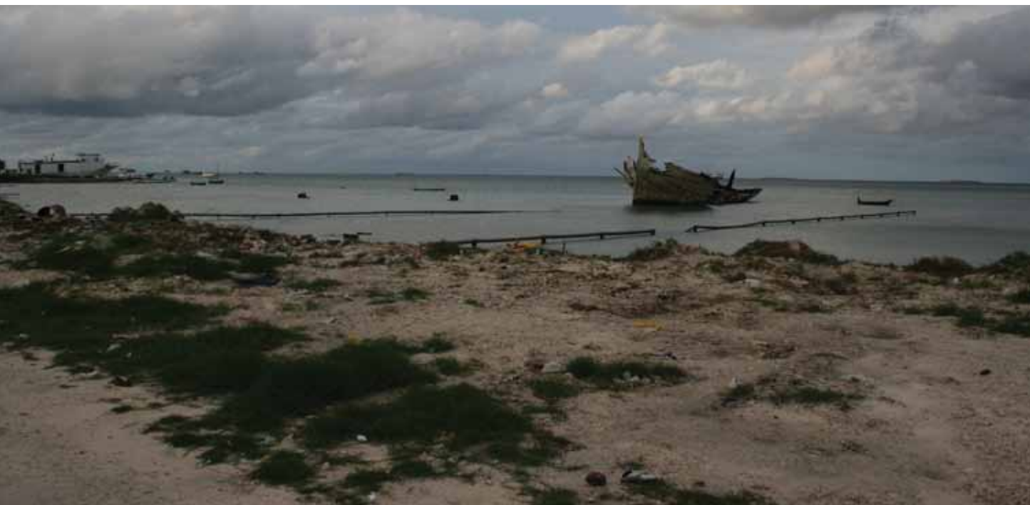
Sewage outlets into shallow water above the coral reef on Thinadhoo
