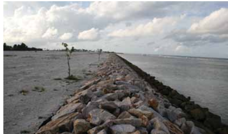
Newly reclaimed land on Viligili showing the uniform height and straight line of the sea defence, combined with a lack of vegetation or 'environmental protection zone'. The original natural island is visible to the left of the picture, where vegetation is established. The reef edge is visible to the right, where the waves are breaking, indicating the increased exposure of the new land.
