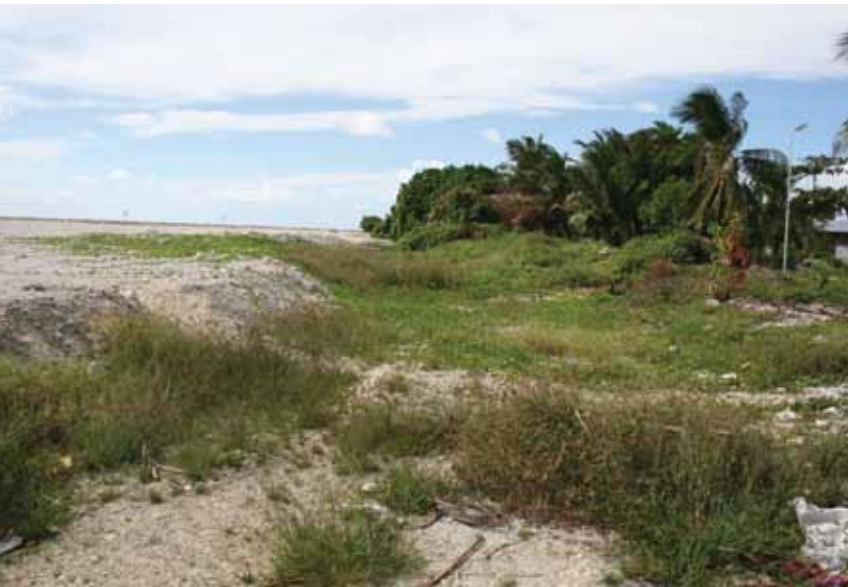
Drainage channel on Viligili next to reclaimed land (on left)
