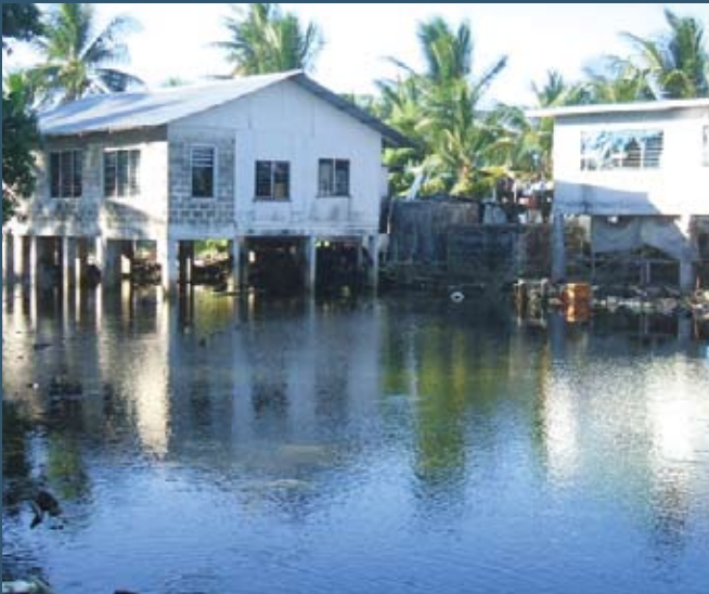
Vanuatu houses built off the ground to avoid flooding. Photo: Shawn Shen.
