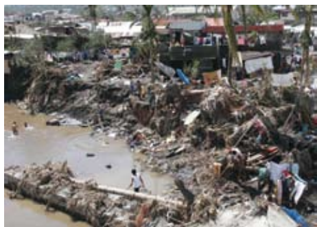
Houses by a collapsed river bank lie in shambles after strong winds and rain from Typhoon Reming battered Legazpi in Albay, Philippines, 340 kilometres southeast of Manila. The latest extreme weather disturbance to hit the country is a portent of more violent weather events that countries around the world are likely to experience in the future as a consequence of climate change. Photo: Ivan Sarenas/Greenpeace.
