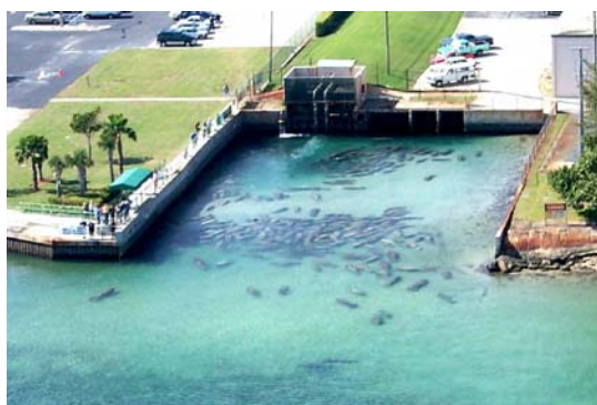
Fig. 3.3: Power plant discharge canal (FWC Manatee Program n.d.)
