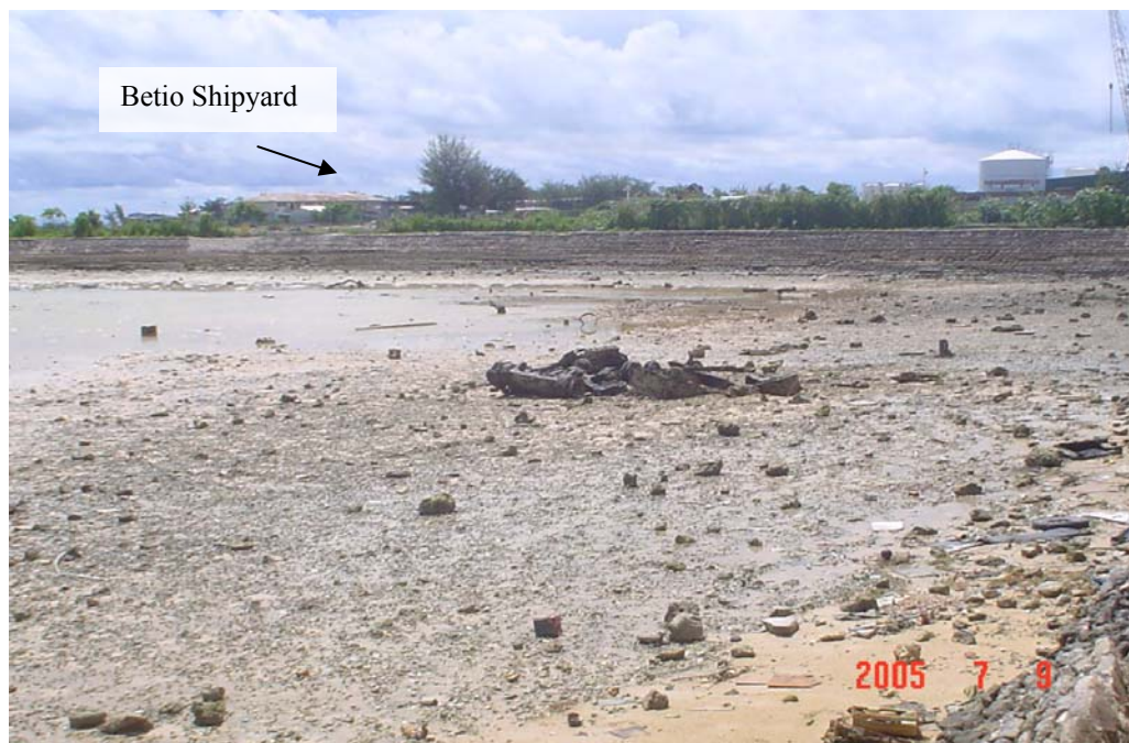
Figure 3.6: Landfill seawall built in 1997 looking into the landfill.
