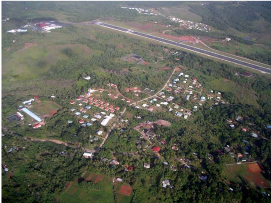
Figure 15. Housing development south of the airport that is experiencing problems with operation of septic tanks, due to the low permeability of the soils in the area (Source: Bob Gavenda, USDA-NRCS Pacific Islands Area).
