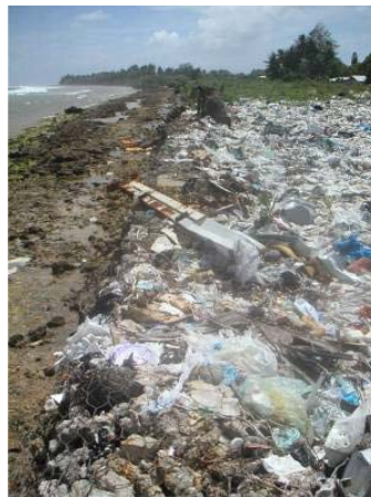
Photo 5-7 Shore protection of the landfill site
