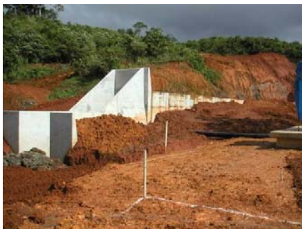
Photo 3-9 Box culvert in the landfill area
