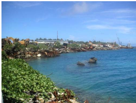
Photo 5-14 Landfill site stretching into the ocean due to discarded vehicles and rubble
