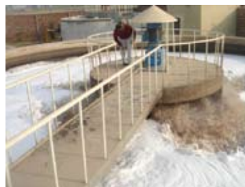
Secondary treatment of tannery waste water
