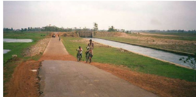
Combining flood management and recharge using the road as a spillway in Orissa, India
