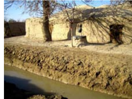
Wells constructed next to irrigation channels in areas with saline groundwater. The wells tap the seepage from the irrigation canals that is less salty, Afghanistan
