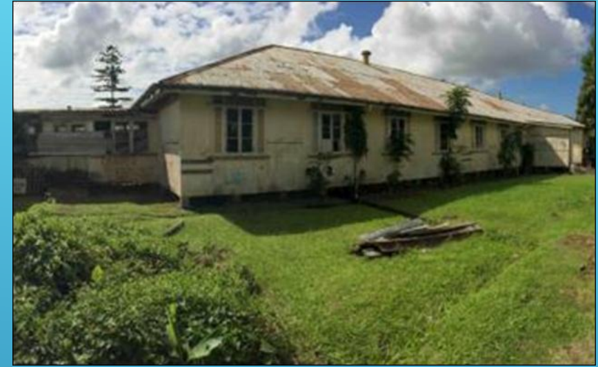
Old Ward 5 Tamavua Hospital Suva
