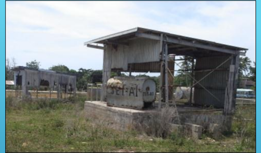
Former Bulk Fuel Terminal, Vava'u
