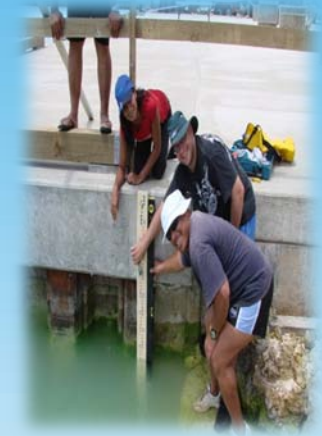
Tide Gauge Installation
