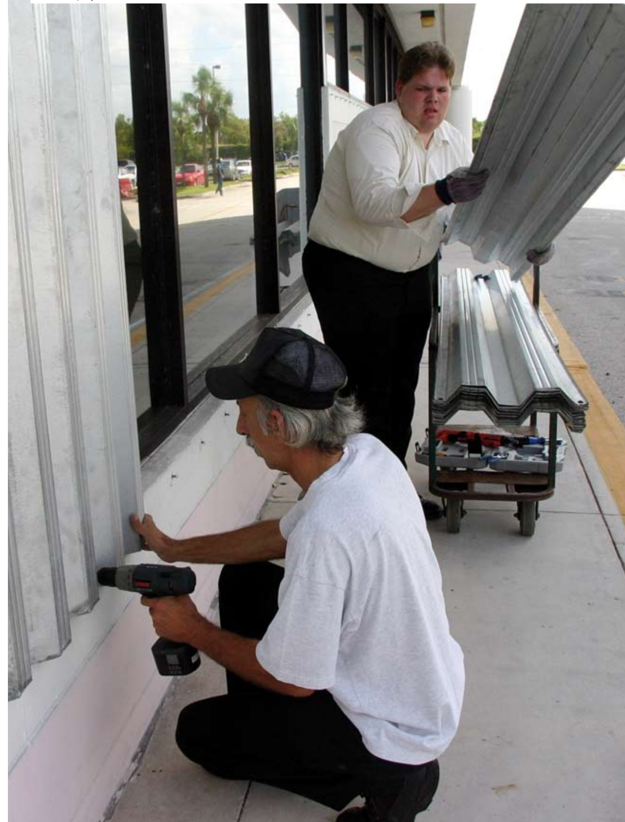
Store employees install shutters for Hurricane Jeanne in Florida, USA. Photo: Reuters/Marc Serota
