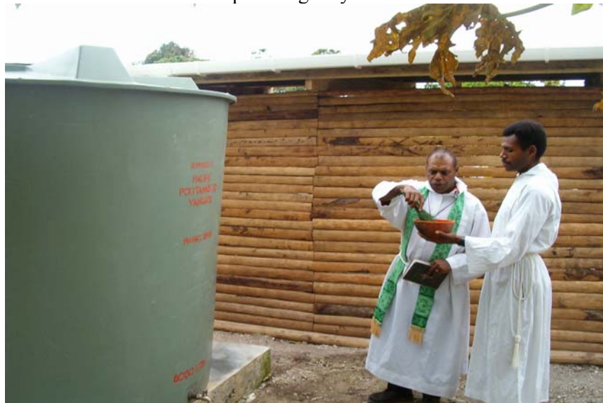
Plate 9 Father Siota sprinkling holy water on the water tanks
