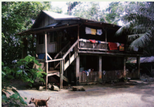
Coping strategies already in use in the Sapwohn study area: a raised external threshold (above) and elevated living areas (below).
