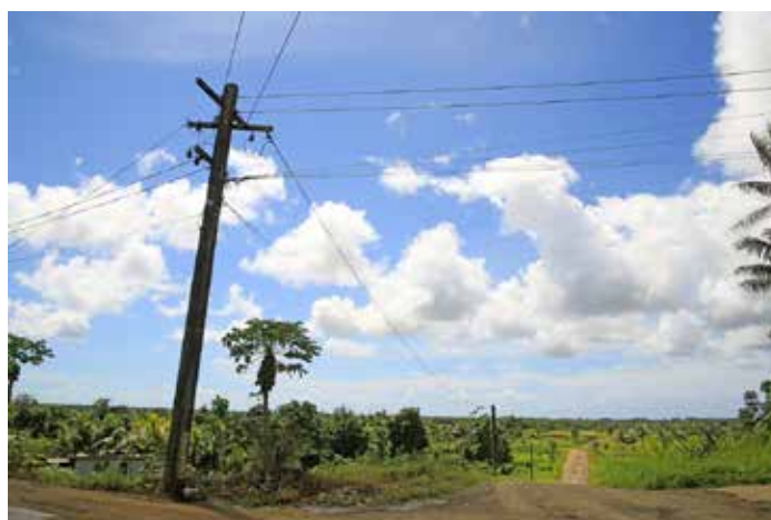
Power lines in rural Fiji (World Bank - A. Nacola)
