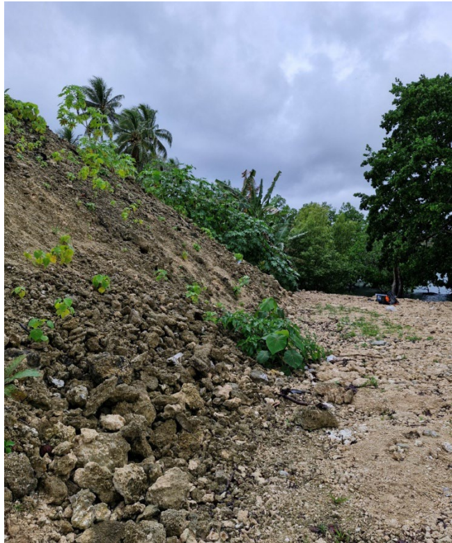
Figure 78. Coastal inundation mitigation measures such as this 10 m sea wall constructed to reduce the impact of sea-level rise to homes and businesses on Santo, impacts natural mangrove functions by hindering tidal inundation, reclamation and natural stratification.
