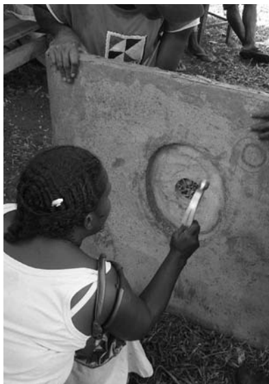
32. Floa slab: Rimuvum fomwok from floa slab. Kilkilim plang blong hol sloslo.
