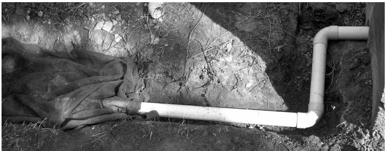
Filta klos i kavremap paep mo ol ston mo i redi blong bakfilim.
