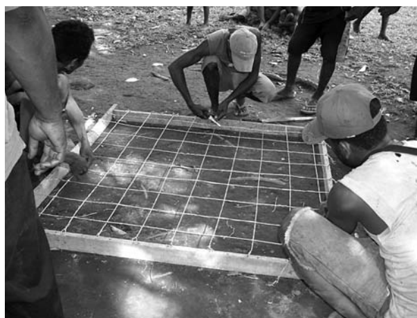
Building the formwork for the toilet slab.
