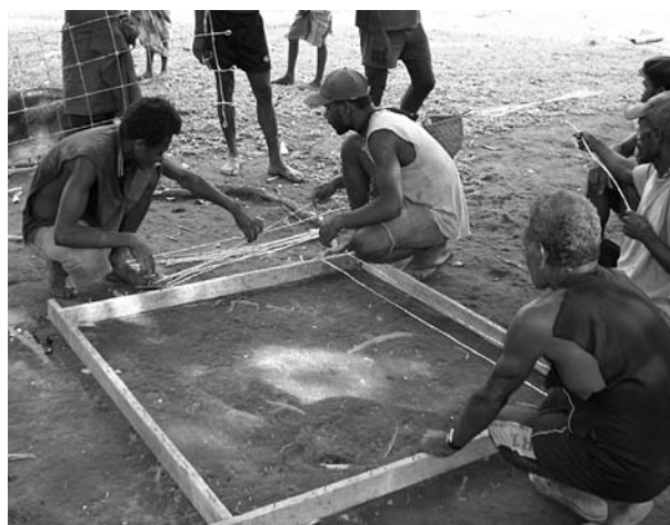
Building the formwork for the toilet slab.
