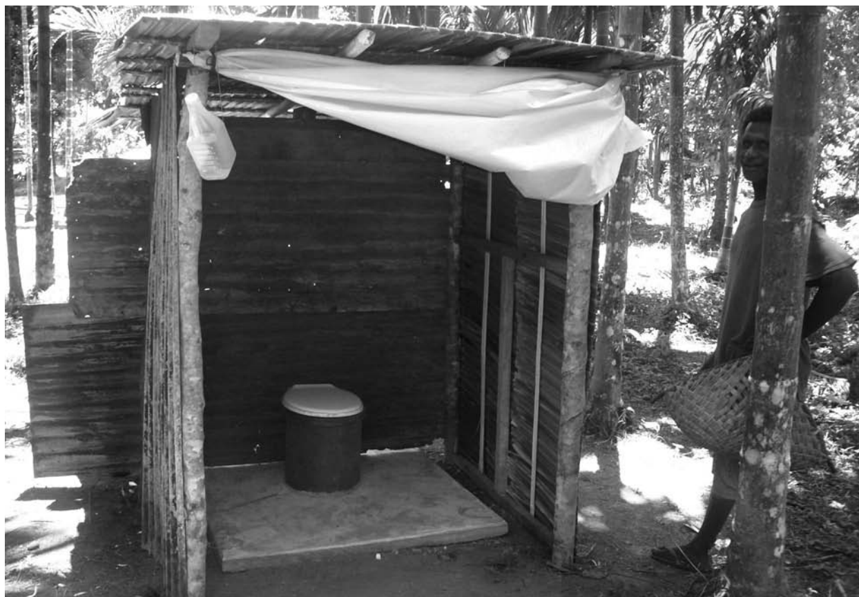
VIP toelet wetem sit raesa long vilij blong Minda, PNG. Win paep bihaen long wol blong bak blong haos hemi pulum moa san mo hot ea blong givhan long ventilesen.
