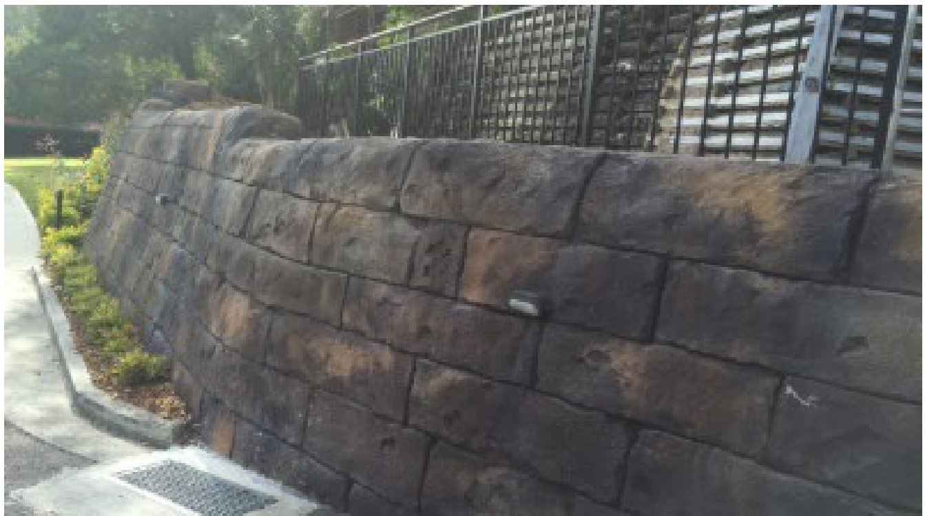
Figure 7: Tire retaining wall covered in sprayed concrete (Tire Stewardship Australia, 2016).
